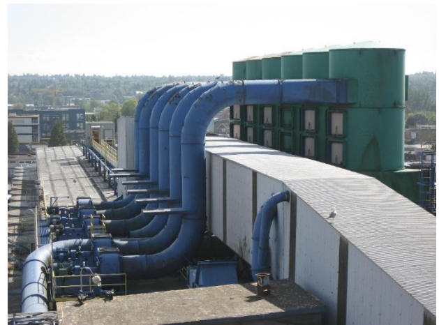
Figure 1: Dust Collectors at a Grain Terminal Facility
