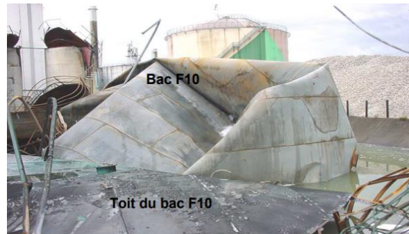
Figure 2 – Bioethanol Storage Tanks After Explosion
